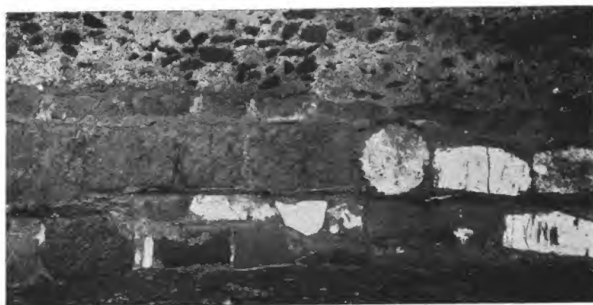
Fig. 153 — S. Lorenzo in Lucina. Foundations of inner lining wall of the apse (Photo: Sansaini).
